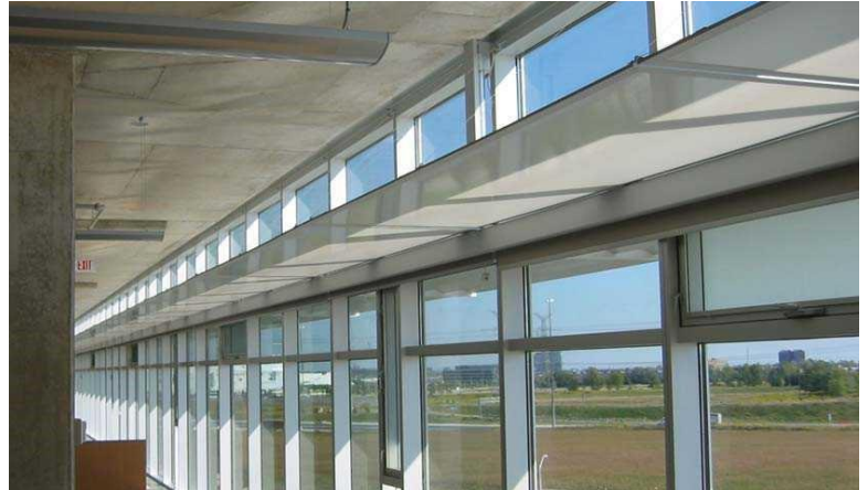
Viewed from the interior, a photograph of a light shelf within a window assembly in the horizontal position. The exterior louvres are in the same plane and partly visible. A rigging system raises and lowers the light shelves and the valence of the window coverings in response to late, low afternoon sun penetrating the building. Loblaw Companies Limited facility designed by Sweeny Sterling Finlayson & Co Architects Inc.
